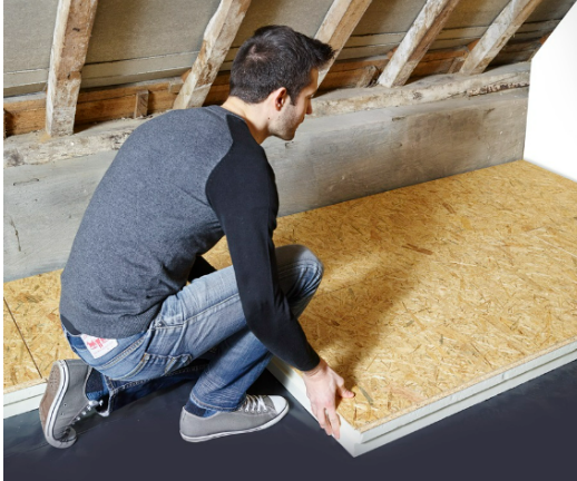
FIGURE 23: COMBINED PU - OSB ELEMENTS
