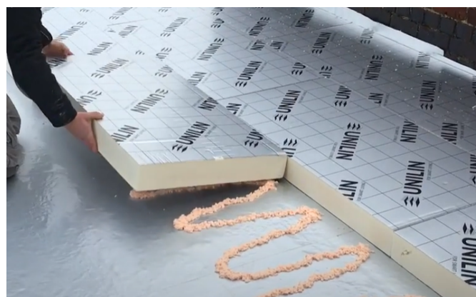
FIGURE 18: GLUING INSULATION BOARD WITH PU COLD ADHESIVE
