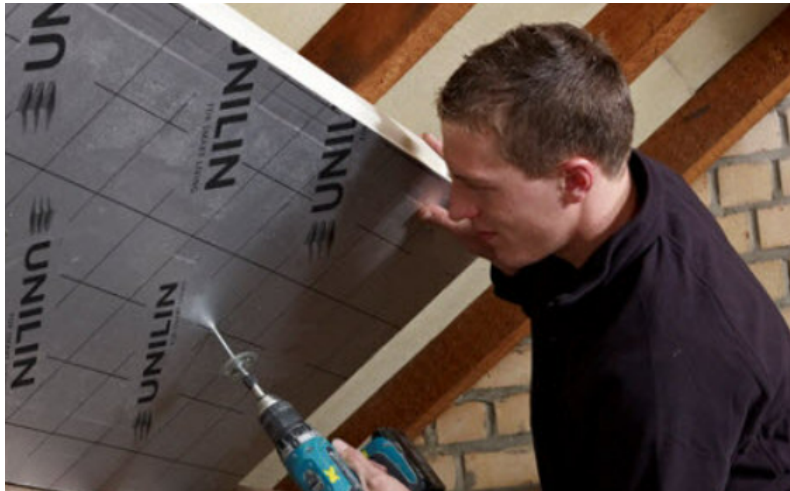
FIGURE 21: INSULATION BOARDS AGAINST THE RAFTERS
