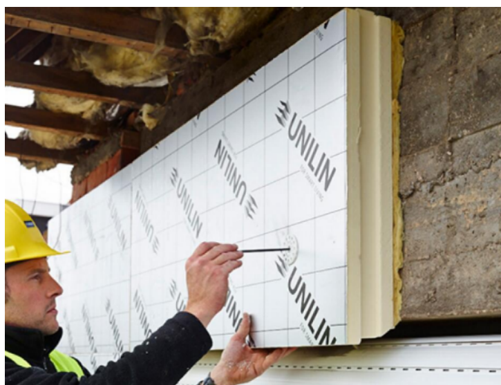
FIGURE 10: INSULATING UNEVEN WALL
