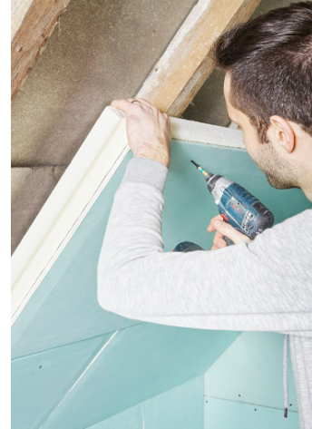
FIGURE 22: COMBINED PU - DRYWALL BOARD
